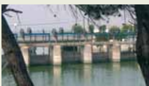
The lock gates
